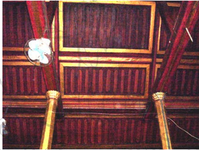
Reception Hall Ceiling of Kyaung Ni Kyaung
