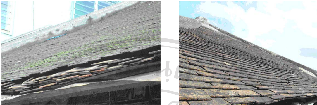
Fig.2.10 The Liet tiles on Ruong houses (left) and on Tu Giac houses (right).
