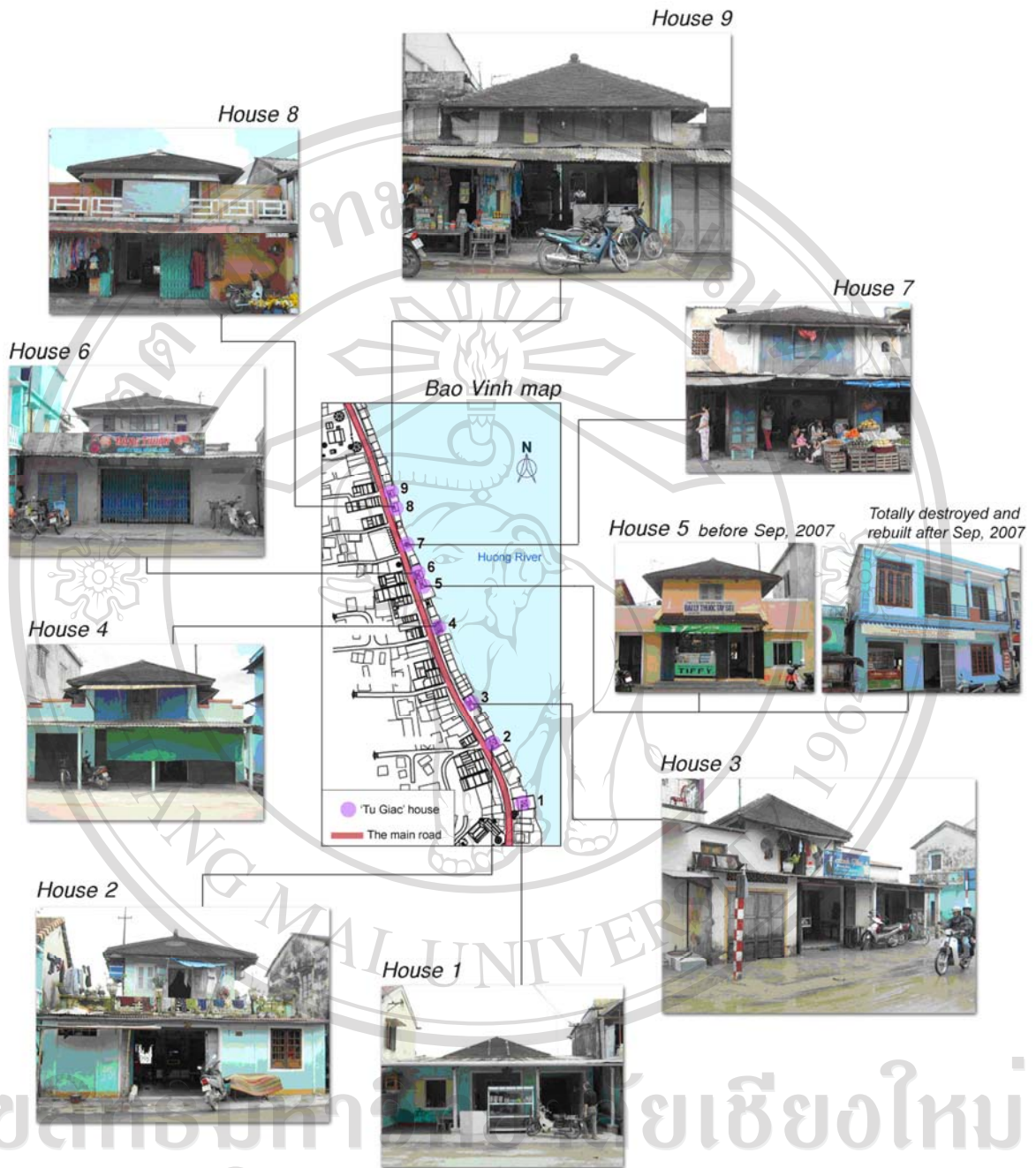
Fig.2.6 The 9 Tu Giac houses on the riverside in Bao Vinh village. House No.5 had been demolished in September of 2007.
