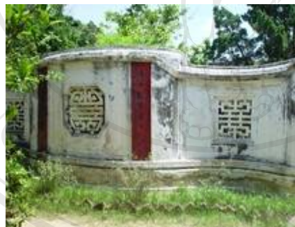
Figure 3-26: The brick screen
